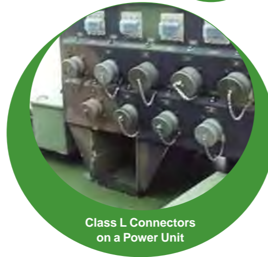
Class L Plug and Receptacle
