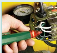
Control panel troubleshoot
