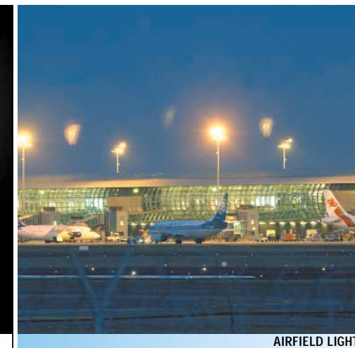
AIRFIELD LIGHTING - TWINARC
