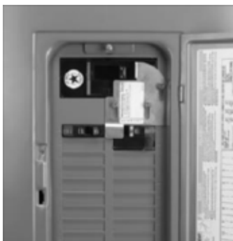
Generator Interlock Kit Installed
