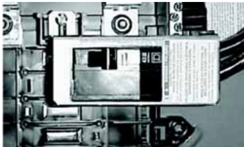
Back-Fed Main Circuit Breaker Retaining Kit
