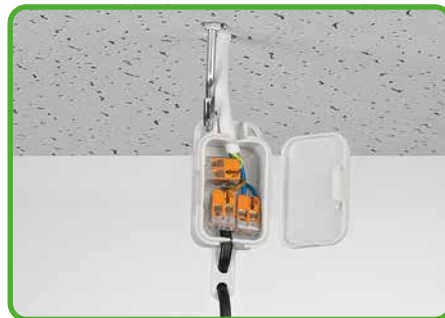
Pendant light connection in suspended ceilings
