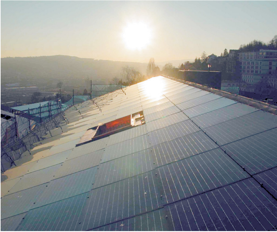
Anlage Application Application Waidspital, Zürich (CH)
