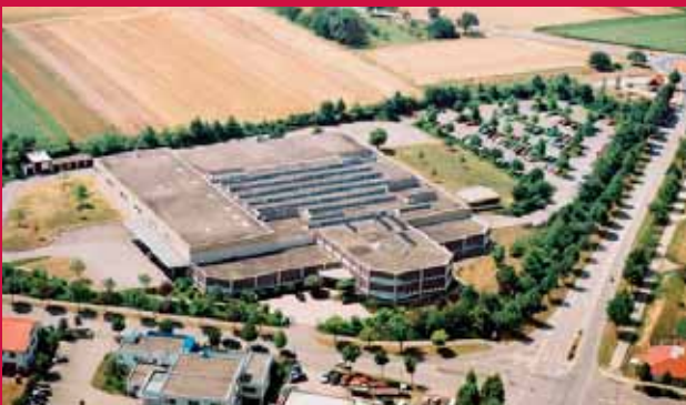
Cooper Hand Tools Besigheim, Germany
