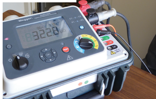
DLRO100H testing rack-mounted, 3-phase circuit breakers
