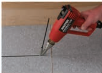
Welding Flooring Material
