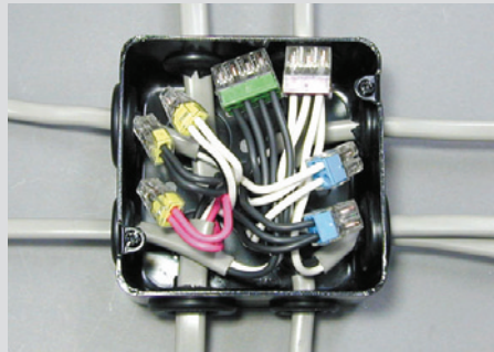
Push-wire connectors used in a junction box. (Japan)
