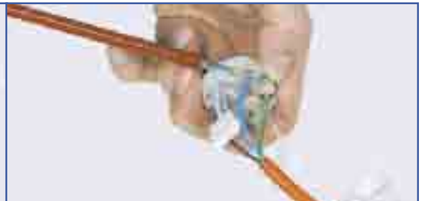
2. Strip Wires, Insert Into Terminals and Tighten Screws
