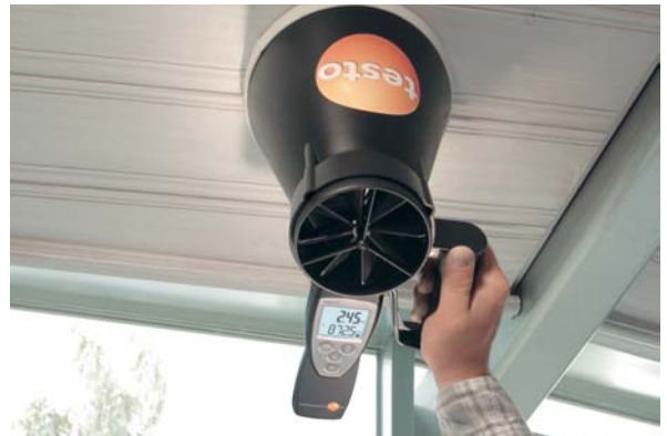
Using the testo 417 to monitor the air input at a ventilation outlet
