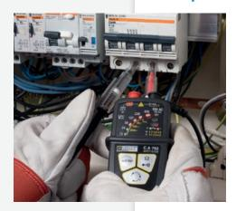
Simple and quick, phase rotation is a useful function, including for circuits isolated by an isolating transformer.
