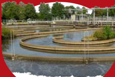
Waste Water Treatment
