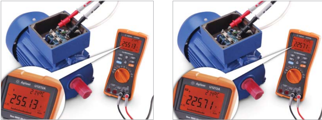
Comparison of voltage output from industrial motor VFD without and with Low Pass Filter functionality.
