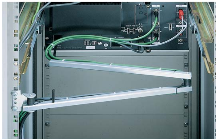
Cable support with return spring
