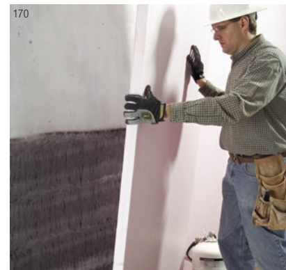
For fast, easy foam board installation, above and below grade, simply spray and stick with 3M™ HoldFast 70 Cylinder Spray Adhesive. Bonds foam to concrete, waterproofing, OSB and more without damaging the foam.
