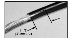
Note: On cables less than 3/4" (19 mm) in diameter, cut a 1 1/2" (38 mm) slit in the sheath opposite connector location. Then complete procedure.
