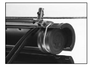
4.02 Remove connector base from bond assembly and insert it between shield and core wrap; inner sheath for double sheath cable, until stops meet outer sheath.
