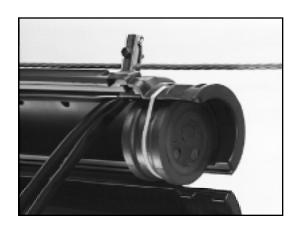
4.02 Remove connector base from bond assembly and insert it between shield and core wrap; inner sheath for double sheath cable, until stops meet outer sheath.
