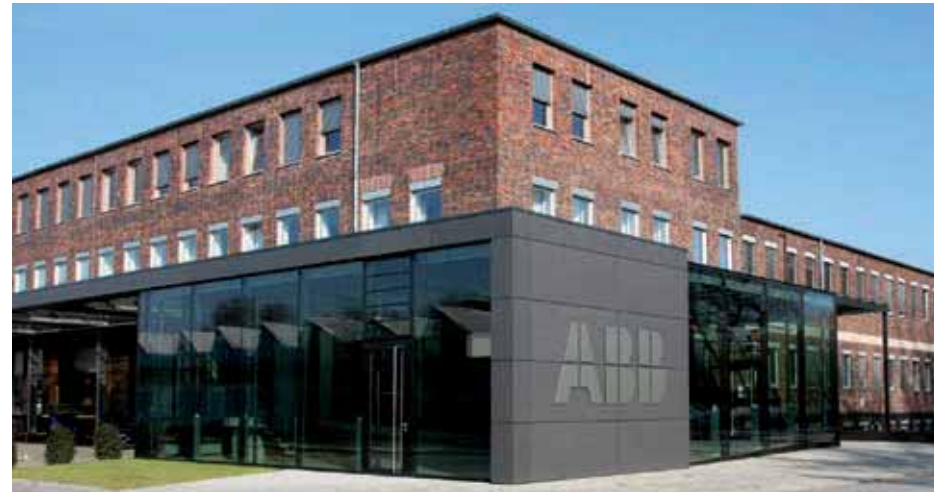
The Stotz Kontakt factory (Heidelberg, Germany)
