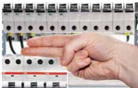
More working space between component rows.
