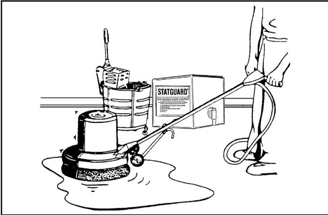
Figure 3. Stripping the floor
