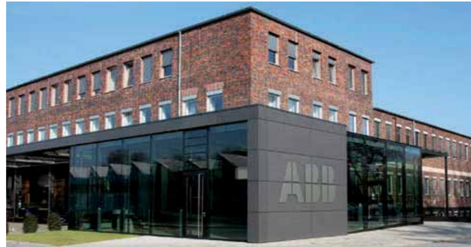
The Stotz Kontakt factory (Heidelberg, Germany)
