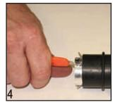
**Step 4:** Remove clear poly interlayer by slitting each end of the tape longitudinally away from the jacket to the end of the cable. Use the inner jacket as a guide to remove each piece of the poly. Do not cut into inner tape. The inner shield will now be fully exposed.
