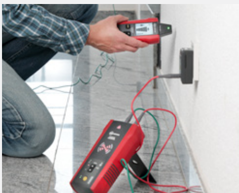
Trace energized and de-energized wires/cables
