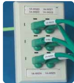
Brady LAT-176-124 is pre-cut for desi-strip inserts in faceplates.
