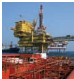
Oil & Gas (Non Hazardous Areas)
