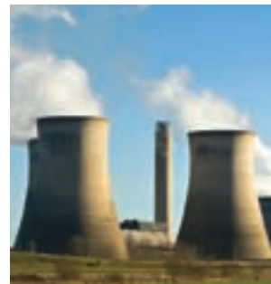
Power Generation & Distribution
