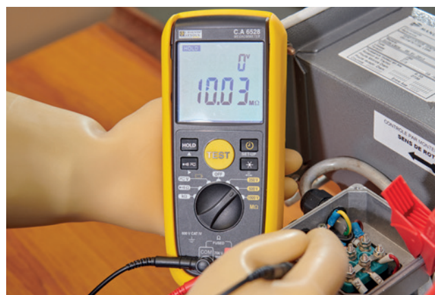
Preventive maintenance on a motor
