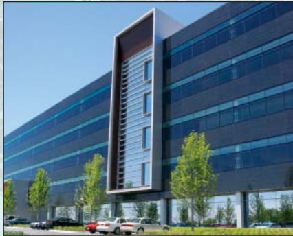
Panduit Corporate World Headquarters Tinley Park, Illinois 60487
