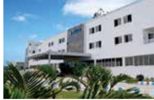
Rudrapur Plant (Green Building)
