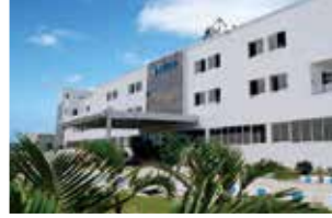
Rudrapur Plant (Green Building)
