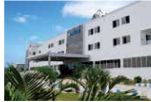
Rudrapur Plant (Green Building)
