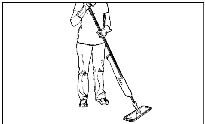
Figure 6. Applying floor finish with Flat Mop (optional)
