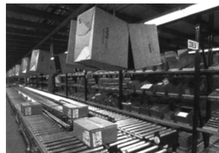
A Limit Switch in Action
