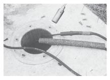
2. Pre-heat cable jacket. Begin shrinking at center, working toward both ends. Use a back-and-forth, sweeping motion of the torch.
