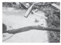
3. Shrinking is complete when melted sealant is squeezed from both ends of the sleeve and all heat-sensitive paint has changed from blue to gray.
