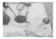
1. Slide the sleeve over cable before making electrical connection. Mate connector sections and wipe dirt from connector and cable. Clean cable with solvent wipe.
