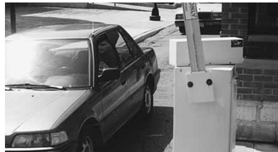
A Photoelectric Sensor Prevents Commuters from Following You Through the Toll Booth for Free
