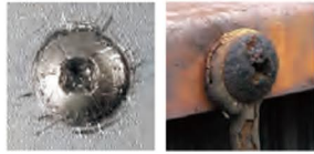
Dome head (Truss)
