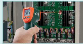
Detect hot spots on circuit breaker panels
