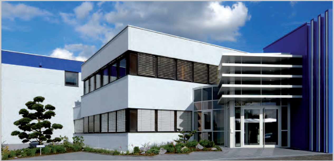
foyer of the company
