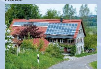
Connected since June 2006: The PV reference system, "Stoiadler III" with 200 modules and 26 KWp of power.
