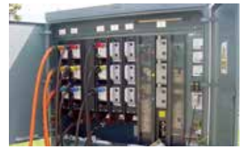
Fuse carriers with integrated PowerLock connectors provide a safe & efficient connection to a power distribution board.
