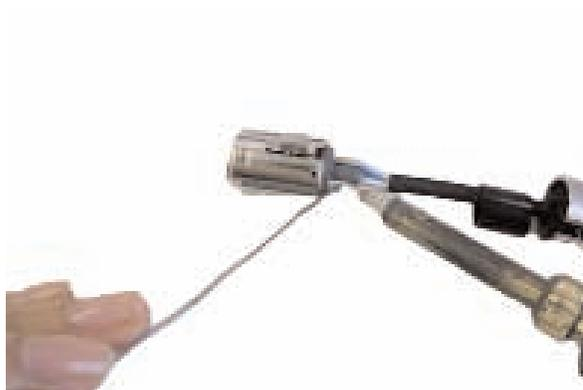
Preparing Insert Assembly; Solder individual center conductors to each contact. Visually inspect solder joints before proceeding.
