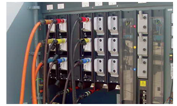
Fuse carriers with integrated PowerLock connectors provide a safe and efficient connection to a power distribution board
