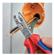
Cutting edges shortening of single wires
