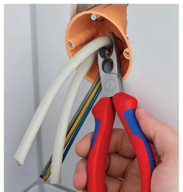
Dismantling deep down in a flush-mounted socket
