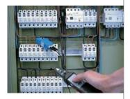
This tracing method uses A1074 current clamps.
