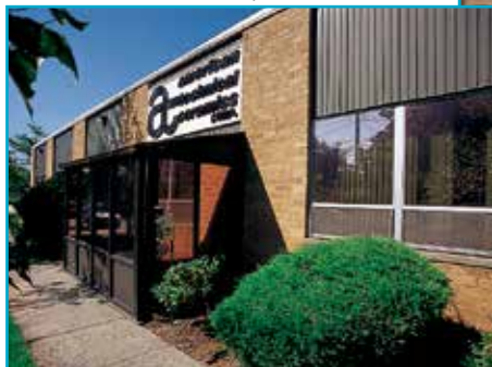
◀ ATC's New York Facility occupies approximately 90,000 sq. ft.
