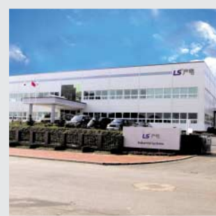
Dalian Plant (China)
