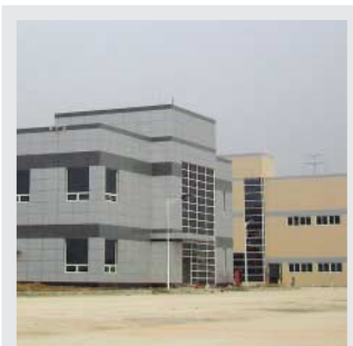
Wuxi Plant (China)
